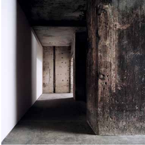
The one-metre-thick walls reveal traces of the bunker's former life / The Feuerle Collection 6
